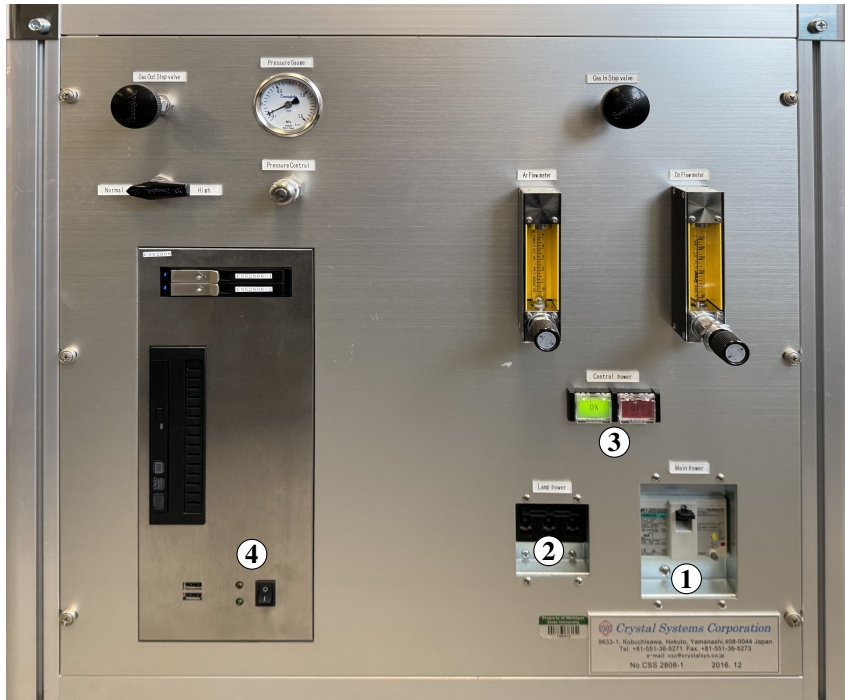
Figure 3: Power switch control panel (call-outs numbered in text).
